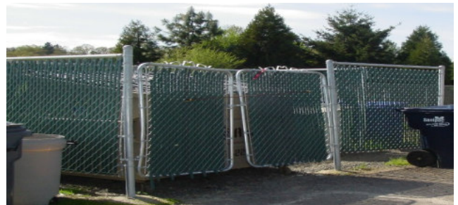
Ryan Salisbury, Troop #97 constructed a barrier for the dumpsters.
